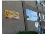
East State Street Center 794 East State St. Trenton
